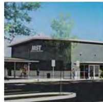
MST O&M Facility Monterey, CA
